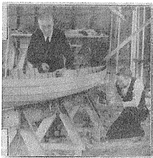
James Greenland and Harry Lounder at work on a clinker-built four in Lounder's Boatshed, c. 1935
